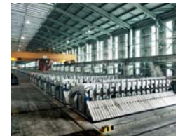
Qatium electrolysis plant, Qatar
